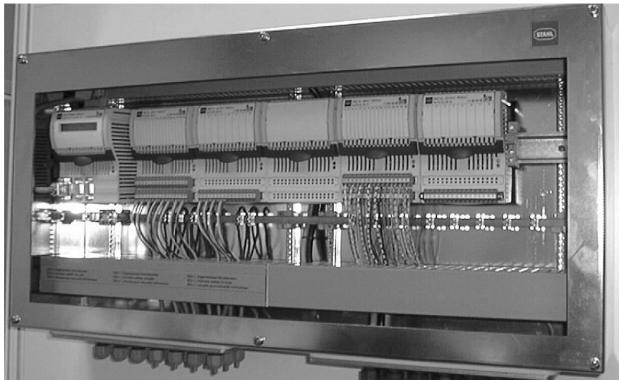
Fig. 4-11 Typical configuration of the I.S. 1 system
