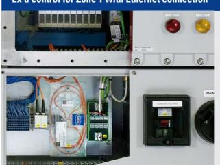
Use of FO splice cassette and Ethernet terminal in the Ex e connection chamber of an Ex d control system.
