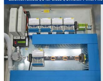
Use of the Ethernet remote I/O system IS1+ in a paint shop in USA with network connectivity via PROFINET protocol.
