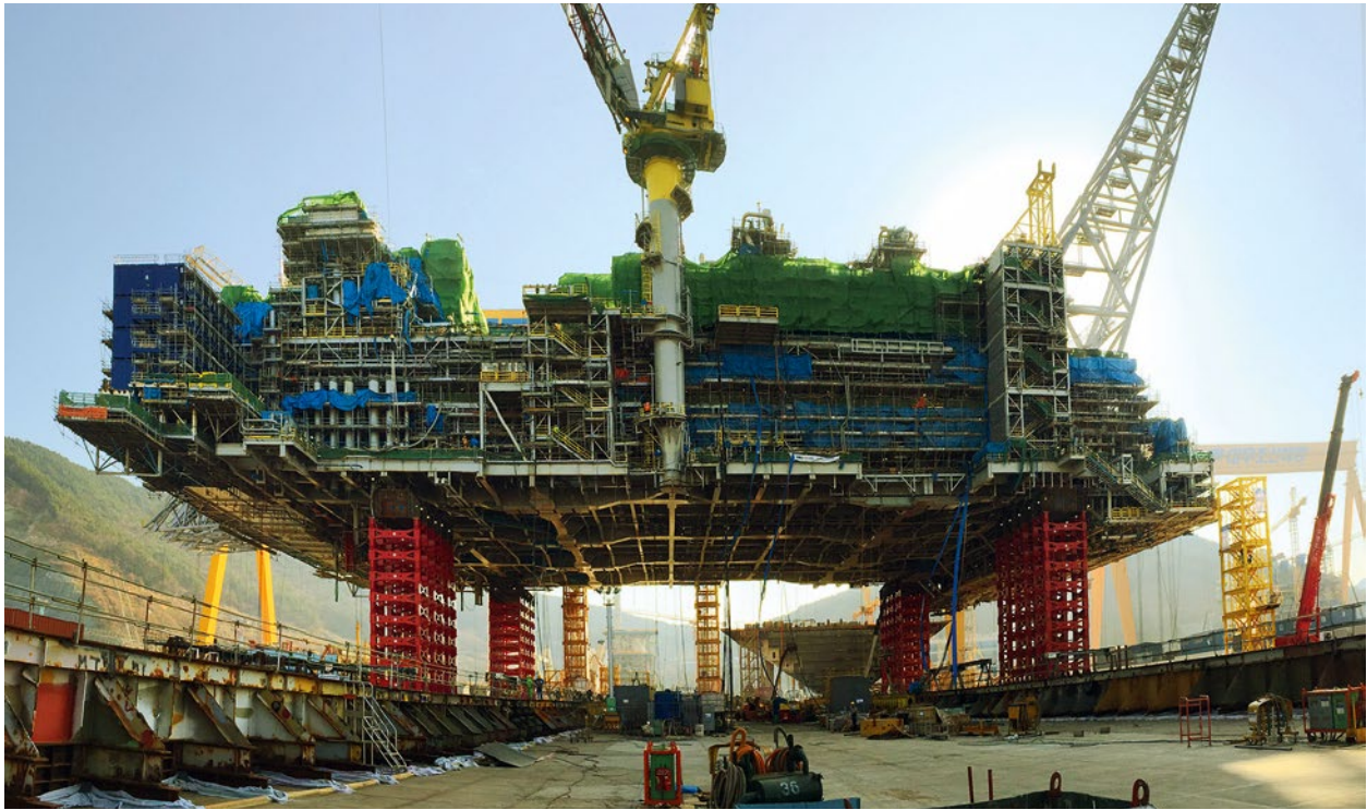
Wheatstone Project in Western Australia
