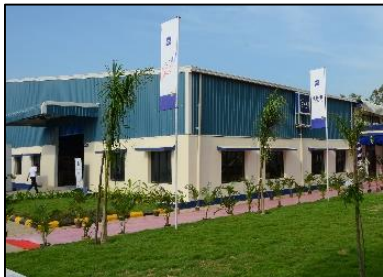
Production site Chennai
